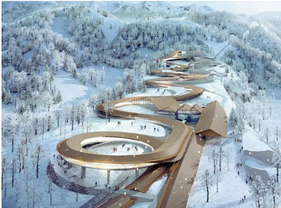
A computer-generated image of the National Sliding Center, which is being built in Beijing's Yanqing district.
